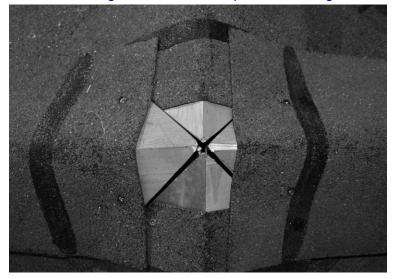
12. Put the top cap in the center of the top cover. See figure below.
