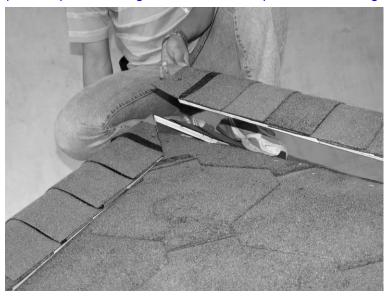
9. Lift the glass fiber tile and fix button of the ridge cover to the top cover by screwdriver. See figure below:
