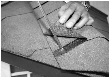
10. Fix another end of ridge cover to the top cover by screwdriver as well. See figure below:
