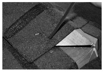
11. Repeat the step 8~10 and fix 4 ridge covers in correct position. See figure below:
